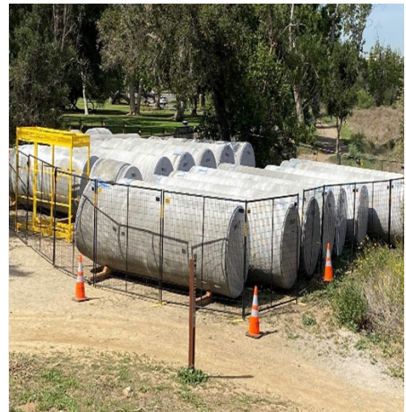
The project included the installation of 54-inch-diameter cement mortar lined and coated steel pipe.
