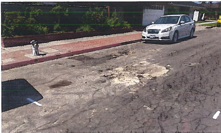
Photo 7: Condition of the pavement within Cameo Highlands, Newport Beach, prior to improvement.
