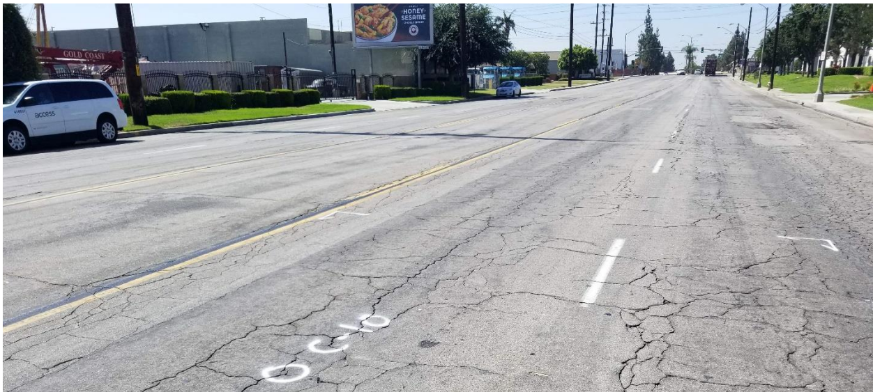
Photo 1: Coring Location C-10, medium- to high-severity alligator cracking, Santa Fe Springs Road, Santa Fe Springs, California
