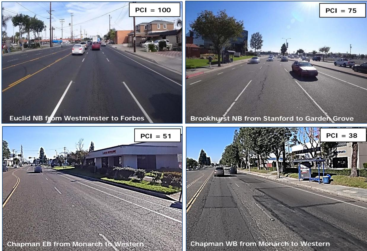
**Figure 1: Pavements with Various PCI's**
