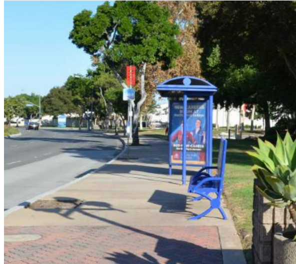
Existing bus stop amenities on Euclid Street, near Acacia Parkway. Bench seating is not situated under bus shelter.
