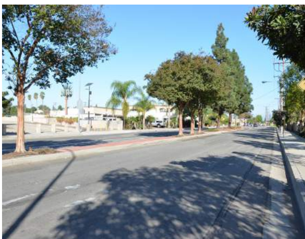
Wide travel lanes present opportunities for traffic calming and accommodation of bikeway facilities.
