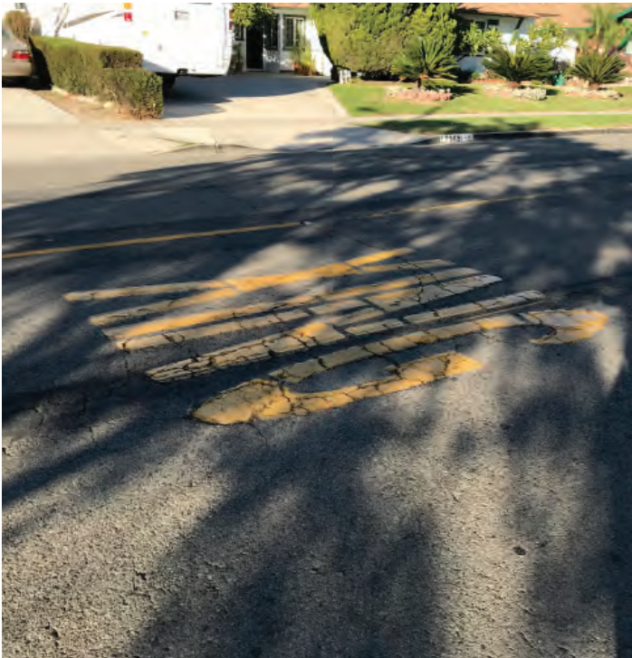
Fading school pavement markings on Woodbury Avenue.
