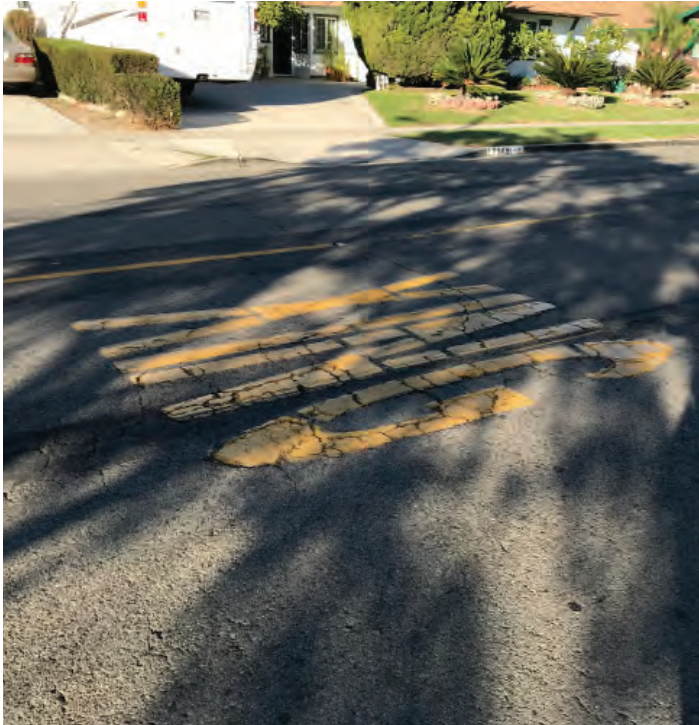
Fading school pavement markings on Woodbury Ave.
