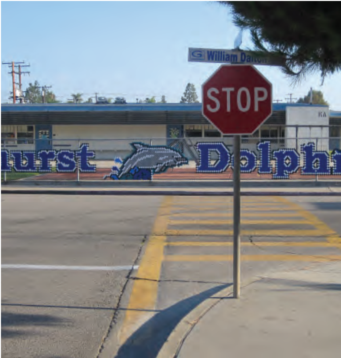
Faded crosswalk & missing curb ramp on William Dalton Way and Hester Place .
