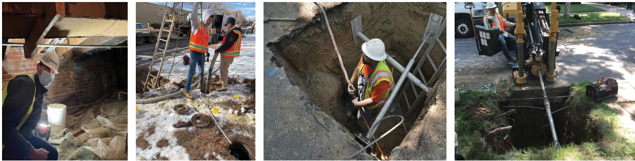
Field Identification and Replacement of galvanized and lead service materials
