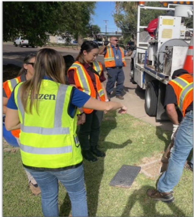
Hazen team members were on-site with Utility staff to test out a utility-owned industrial vacuum truck prior to hiring a third party contractor.
