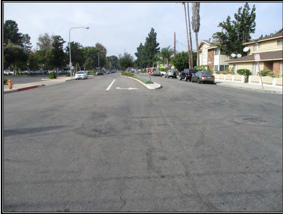
PHOTO NO. 6: View looking west along Stanford Avenue.
