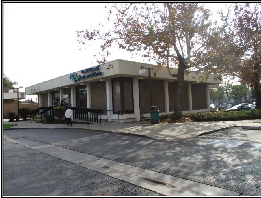
PHOTO NO. 4: View looking southeasterly at the bank facility.
