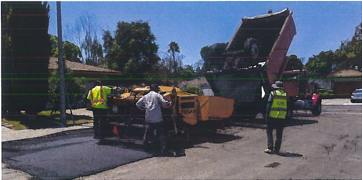
Photo 4: GMU performing observation and testing for Mission Viejo's 2020 Residential Paving project.
