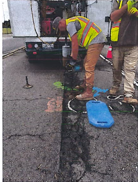
Photo 3: Coring performed on Hamilton Avenue, City of Huntington Beach.
