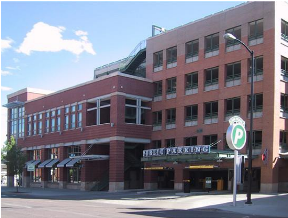
Photo 9.18-9: Example of Parking Structure Architectural Treatment
