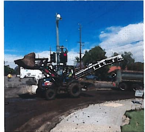
Cold milling on Ontario Avenue, City of Ontario
