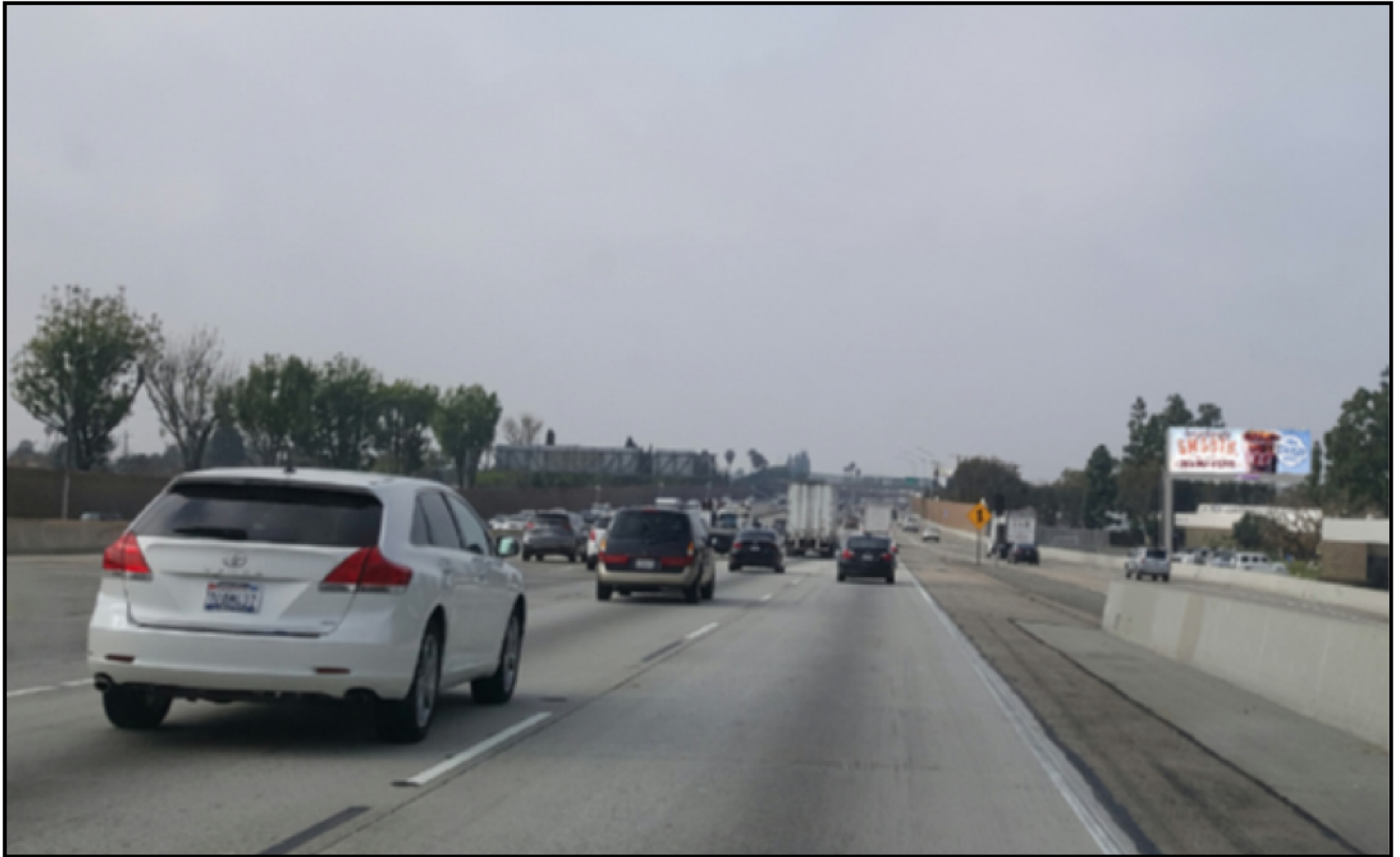
View #1: From Westbound Travel Lanes on SR-22 Freeway (Proposed LED Billboard)
