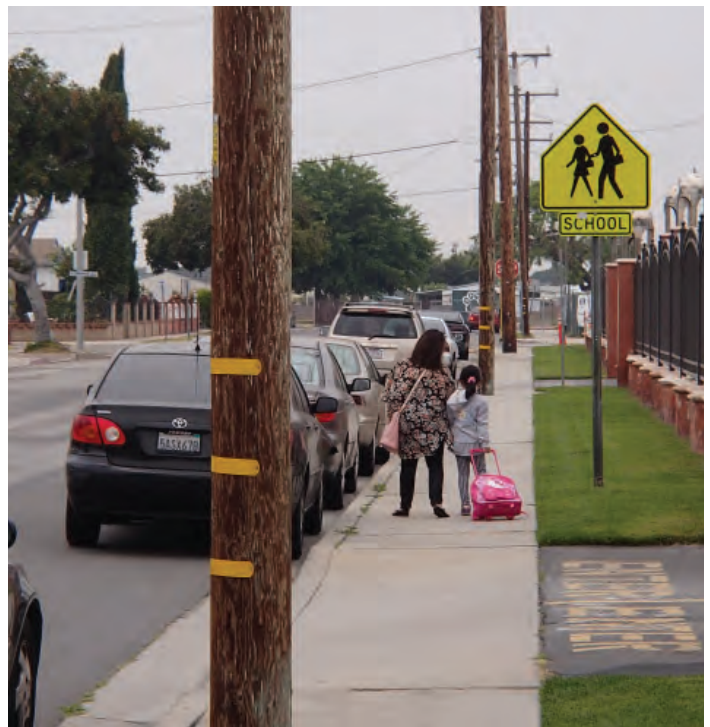
Outdated school signage along 11th Street.
