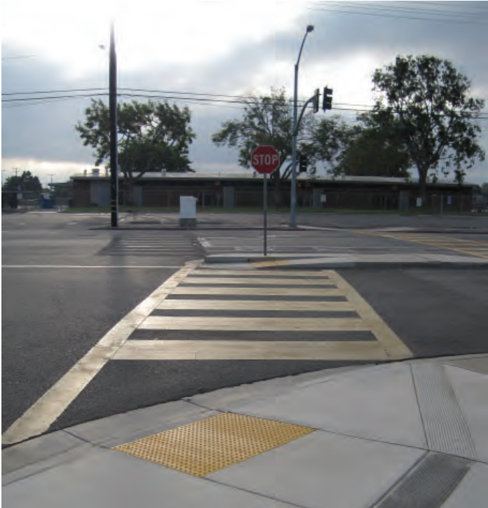
Existing high visibility crosswalk and ADA compliant curb ramps at Florence Ave/Ward St frontage road.
