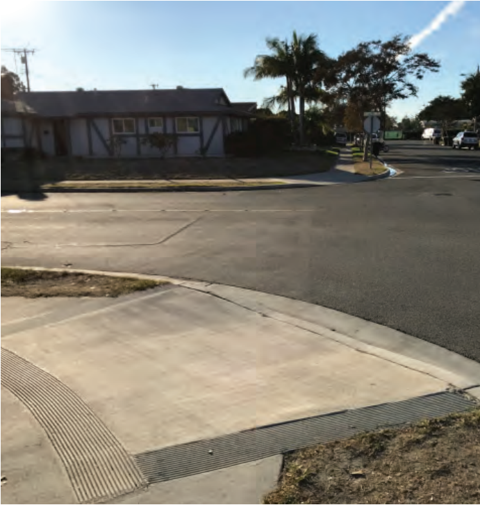
Existing curb ramps at the intersection of Erin Street and Woodbury Avenue.
