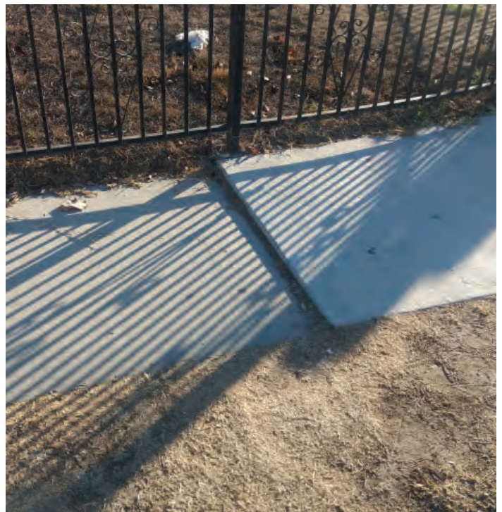
Uneven sidewalk on Woodbury Avenue and various other locations throughout the neighborhood streets.
