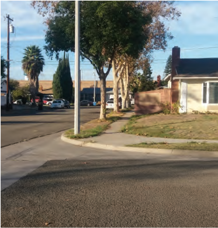
Uncontrolled intersection without curb ramps.
