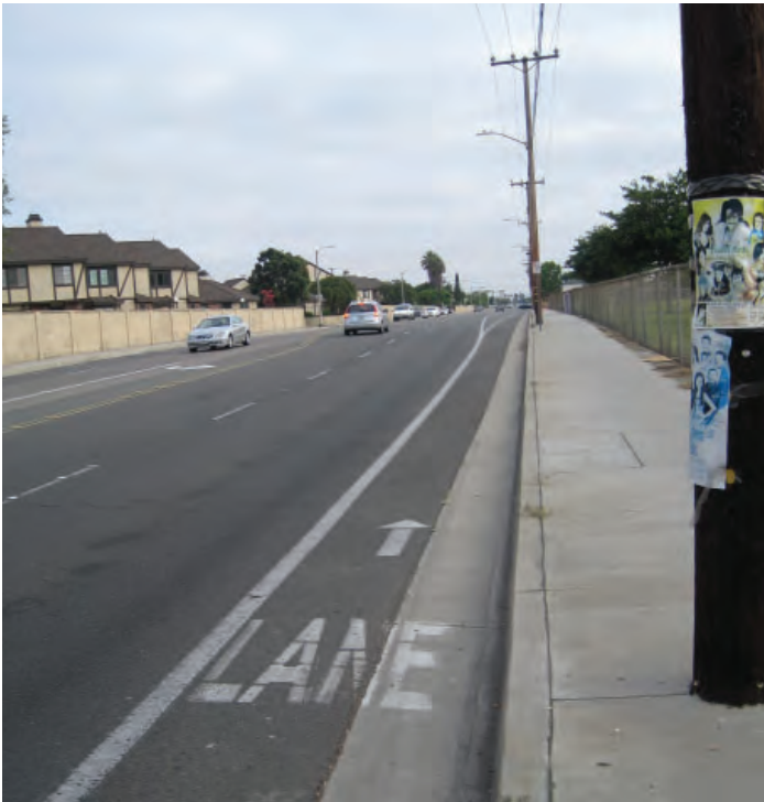
Existing bike lane with two vehicle travel lanes in each direction along Bushard Street adjacent to the school.
