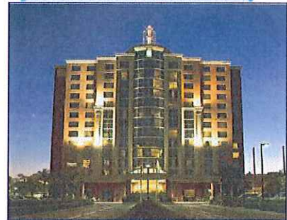
Embassy Suites Hotel in the International West Resort Area
