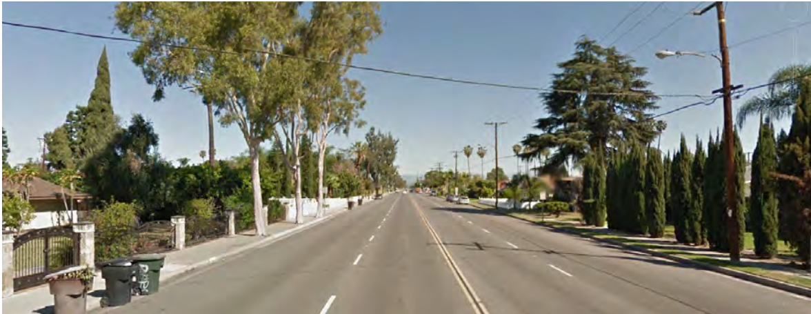
Road Rebalancing. Gilbert Street looking north from Shannon Avenue.
