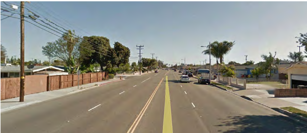
Road Rebalancing. West Street, looking south along residential neighborhood, north of Chapman Avenue.
