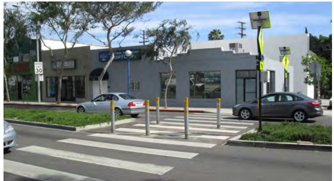
A midblock crossing in West Hollywood, CA features a high-visibility crosswalks, bollards, and flashing beacons for a safe, convenient walking environment
