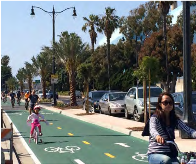
A separated bikeway provides a physical separation from motor vehicles.
