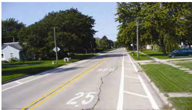
Examples of traffic calming through painted shoulder markings (left) or painted center median (right)
