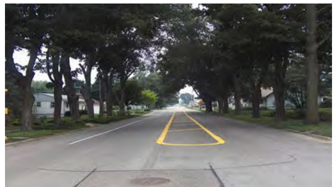
Examples of traffic calming through painted shoulder markings (left) or painted center median (right)
