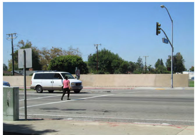
Woman crossing Bixby Avenue. This intersection uses transverse crosswalk striping.
