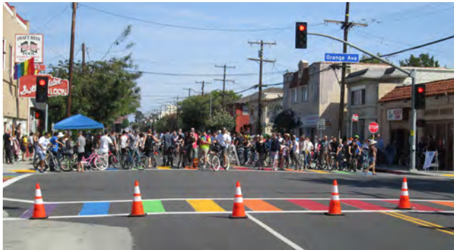
A creative crosswalk in Long Beach, CA provides more visibility and enjoyability for pedestrians
