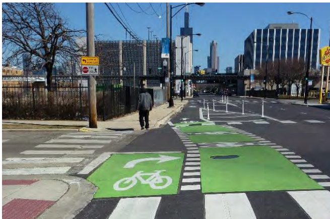
Bicycle-friendly intersection treatments including paint, bicycle signals, and bicycle boxes
