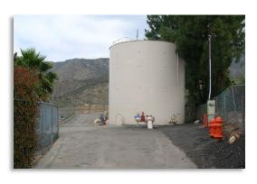
**Phase B** | Miscellaneous piping and appurtenances in Plant 137 were retrofitted. Equipment not connected to the system which include piping, tanks and valves were removed. Any salvageable equipment was reused at other plants. Existing above ground piping and valves that showed signs of corrosion were replaced.
