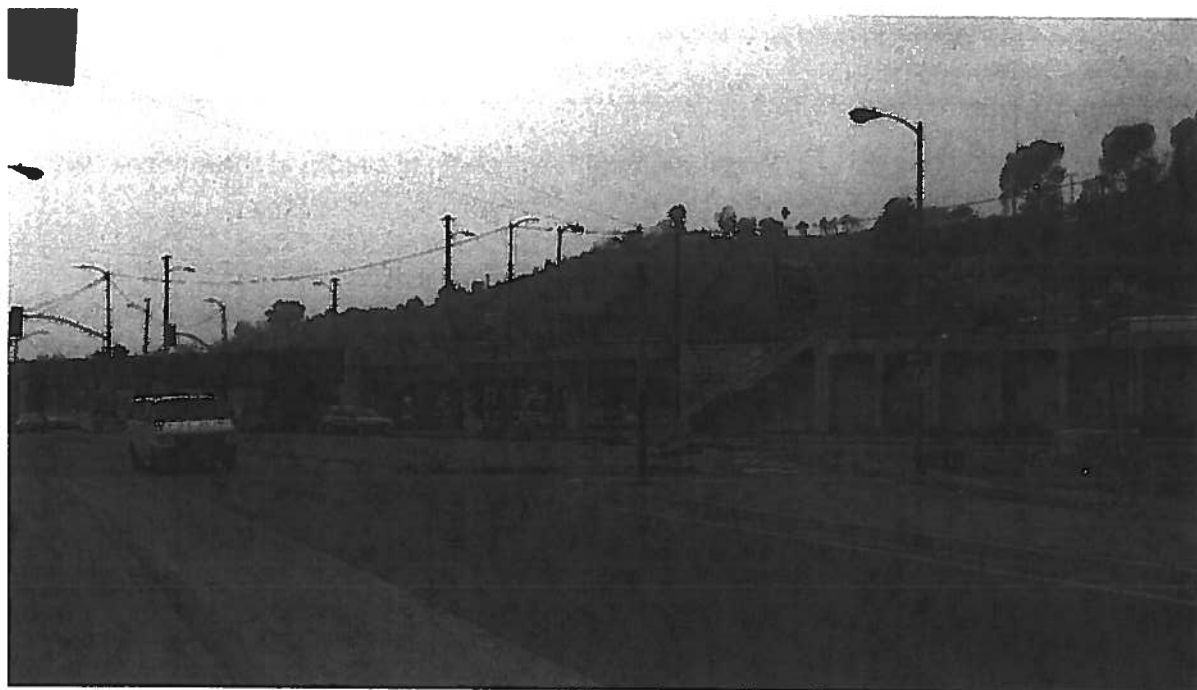
Soto Bridge Over Mission and Huntington Drive-During Stage 1 Construction
