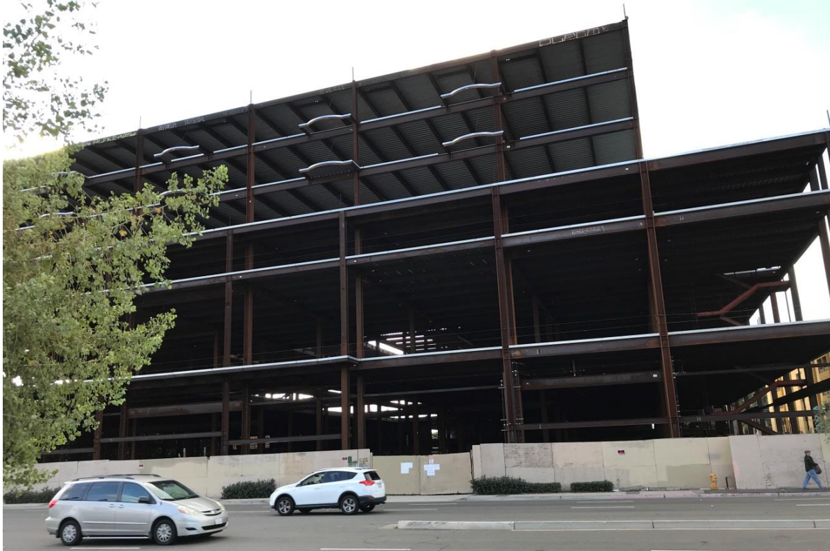
Figure 3a View of Project Site Looking South across Garden Grove Boulevard
